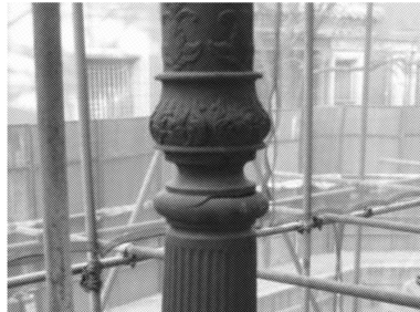
(c) 柱裂缝
